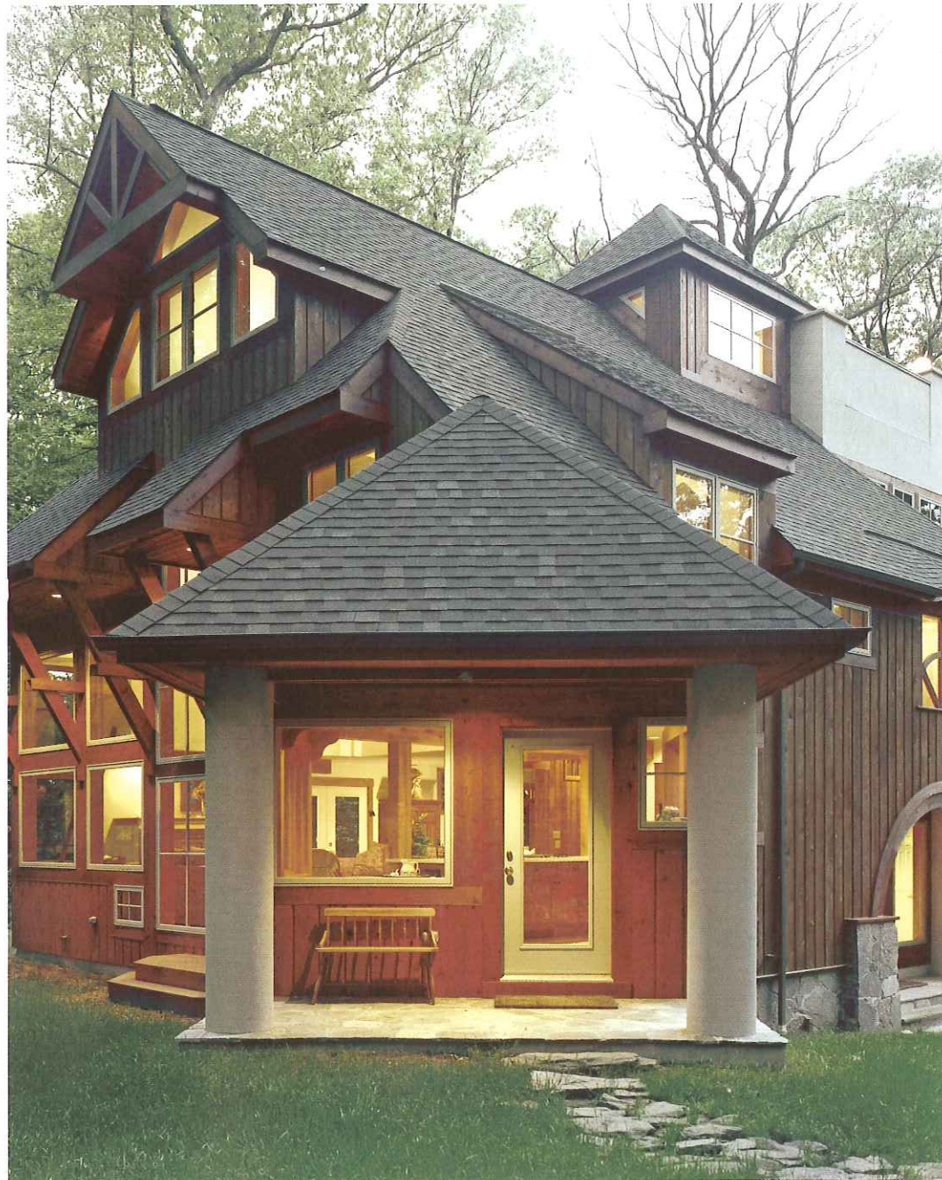
Above: The ultimate "green" home, this is a new 3,000-square-foot super insulated, penalized constructed residence. Use of natural materials throughout emphasizes the relationship to its wooded landscape. Good air quality is insured by introducing fresh air via a heat recovery system. Owners—Regina and Shawn Carey Photograph by Tom Bernard
